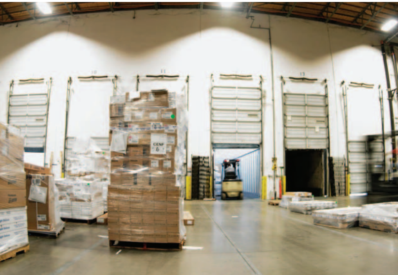
Occupancy sensors and controls, integrated into the fixtures, provide energy savings.
